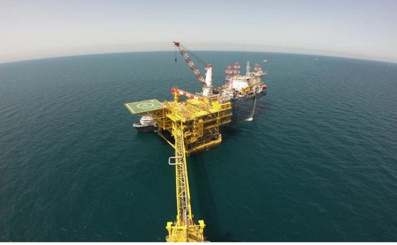
A fully-integrated gas platform - the heaviest in Saudi Aramco's history - installed by float-over method at Hasbah Field in Saudi Arabia
