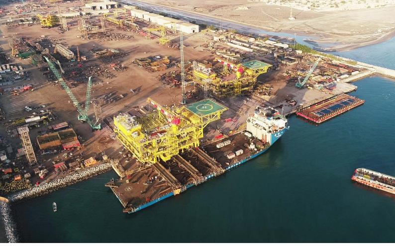
Load-out of two mega Tie-in Platforms (7000 MT each) for Hasbah Field, Saudi Aramco from L&T Hydrocarbon Engineering's Oman facility
