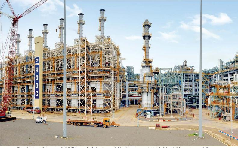
The world's largest ethylene cracker (1.4 MMTPA) – one of multiple systems supplied, installed and pre-commissioned for Reliance's J3 Program, Jamnagar, India. This ethylene cracker is part of ROGC (Refinery Off Gas Cracker), heart of C2 Complex.
