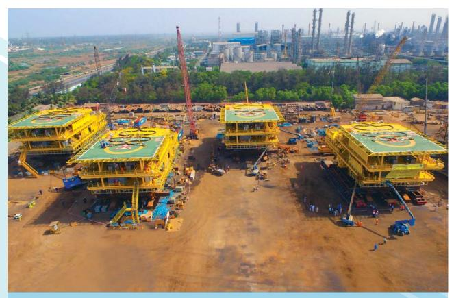
Four Production Deck Modules for Saudi Aramco ready for despatch from Modular Fabrication Facility, Hazira to Safaniya Field, Saudi Arabia
