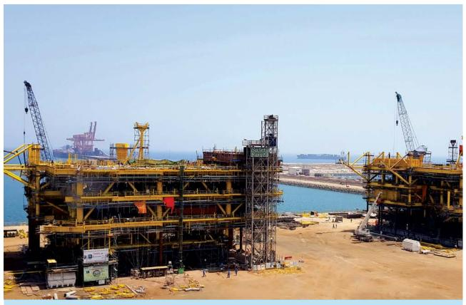
Two tie-in platforms, 7500 MT each, under fabrication at Modular Fabrication Yard, Oman, for Saudi Aramco's Hasbah II Gas Increment Project. The USD 1.6 billion project also includes six gas production deck modules, two six-legged jackets, pipelines, composite cables, umbilical and onshore valve stations.
