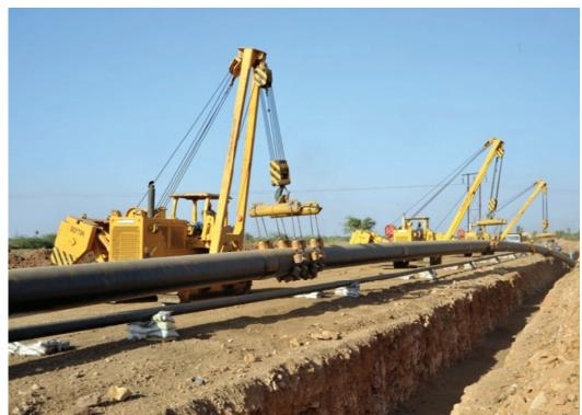
World's Longest Heated and PUF-Insulated Waxy Crude Oil Pipeline fromBarmer (Rajasthan) to Bhogat (Gujarat)
