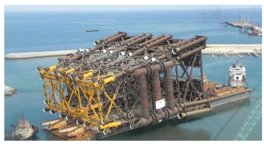
Sail-away of jacket for Asia's largest process platform (13,500 MT, 8-legged launch-type with 23 pre-installed risers) from Modular Fabrication Facility at Sohar in Oman
