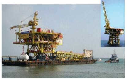
Topside & Vent Boom being transported to Yetagun field (inset: Yetagun D Platform installed Offshore)
