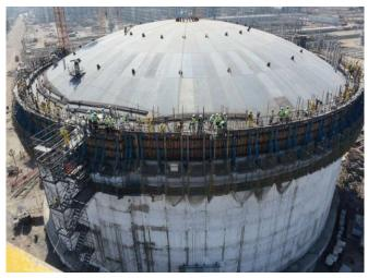
Cryogenic Ethylene Tank – Dome Air Raising
