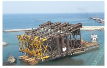
Sail-away of jacket for Asia's largest process platform (13,500 MT, 8-legged launch-type with 23 pre-installed risers) from Modular Fabrication Facility at Sohar in Oman
