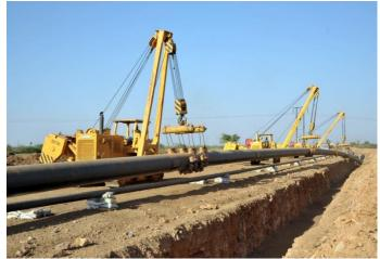
World's Longest Heated and PUF-Insulated Waxy Crude Oil Pipeline from Barmer (Rajasthan) to Bhogat (Gujarat)
