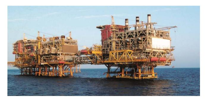
BCP-B2 process platform with an interconnecting bridge built for ONGC
