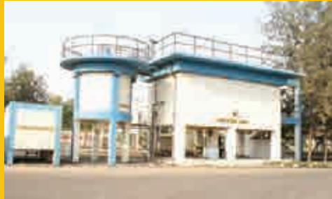
STP at Hazira MFF
