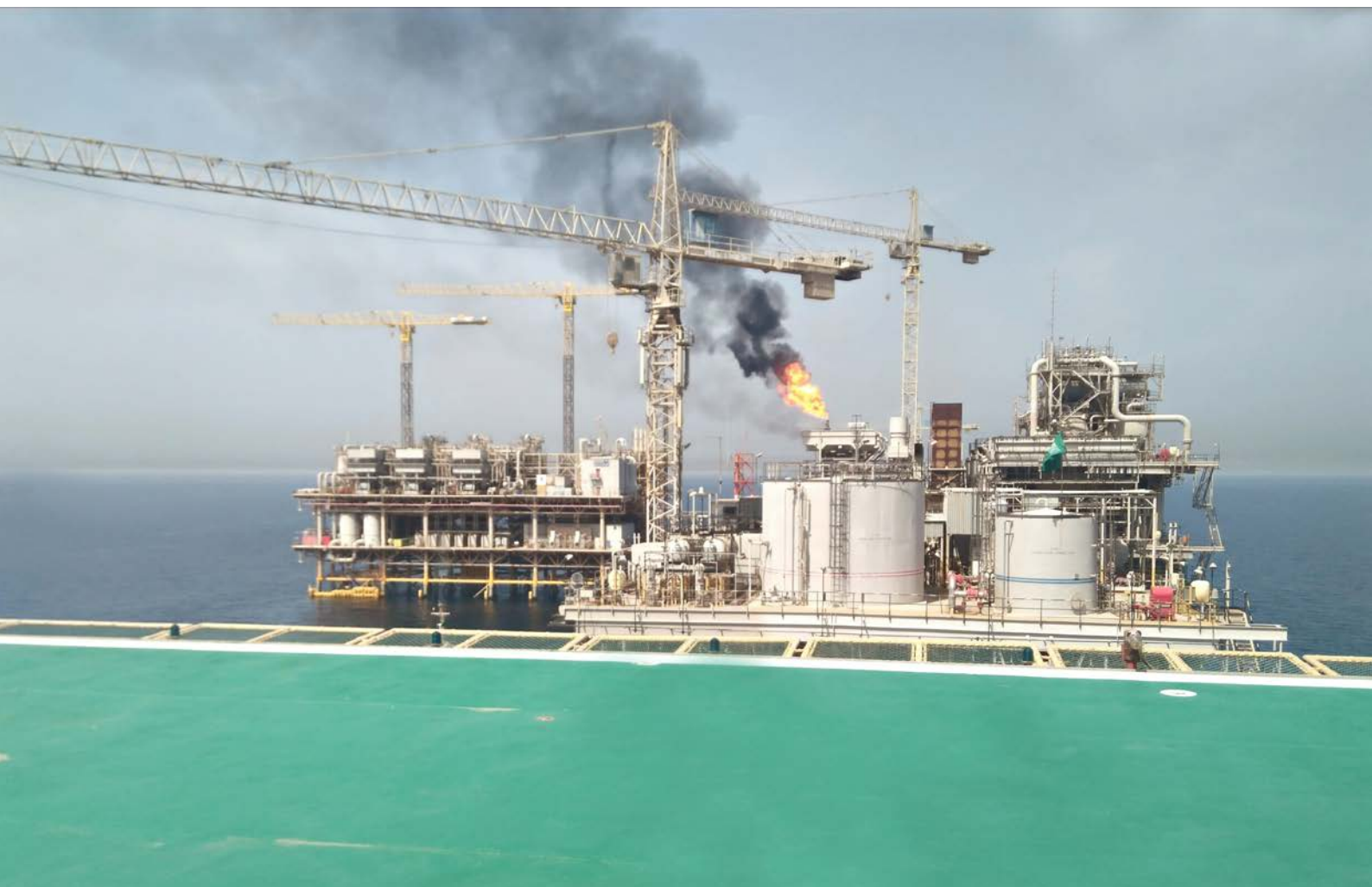
A snapshot of the 17 tower crane replacement project for Saudi Aramco.
