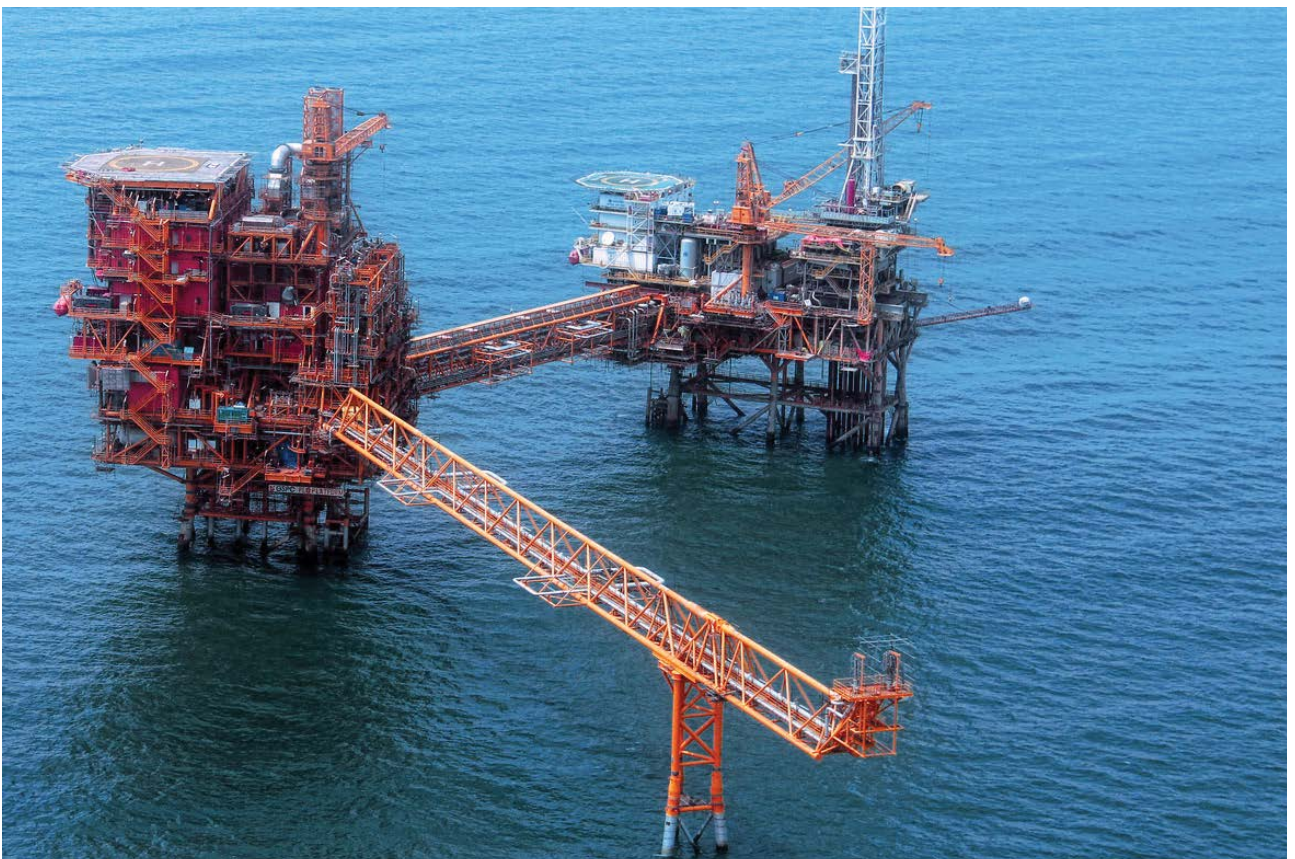
Wellhead platform and Process-cum-Living Quarters Platform installed off India's east coast
