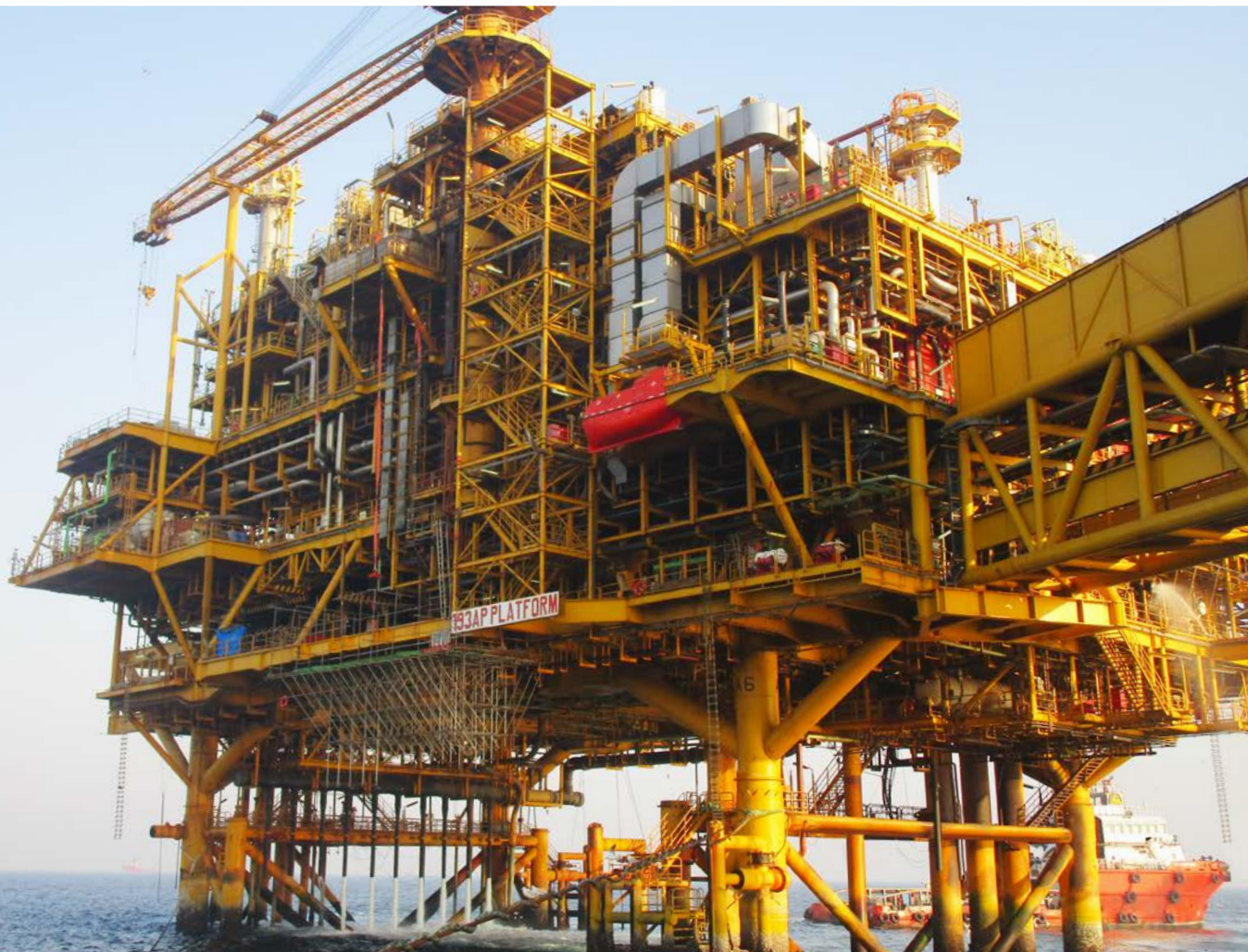
Bassein Development 3 (BD3) Well Platform & Pipeline Project for ONGC
