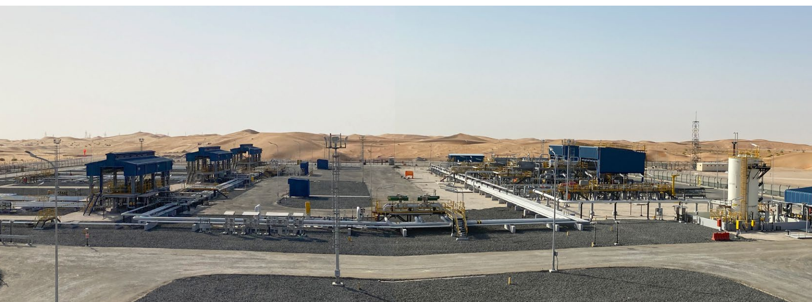
Haliba Field Development Project for Al Dhafra Petroleum Operations Company, UAE.
