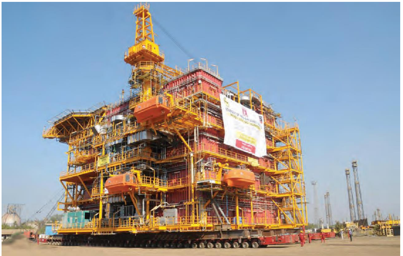
Load-out of India's heaviest module (5300 MT), 150-man living quarters for ONGC, India
