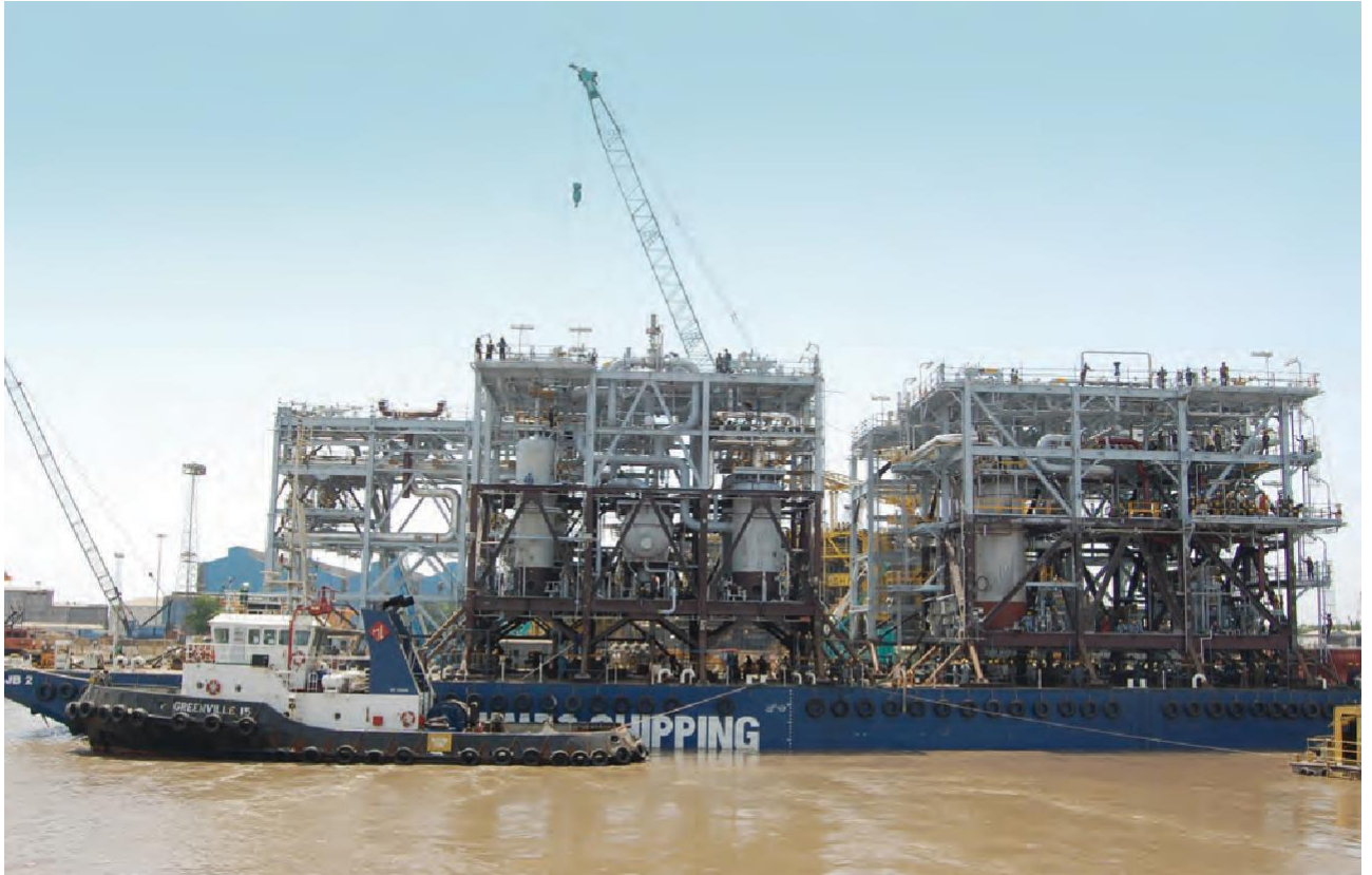
Onshore processing modules (8 Nos.) for ADGAS-OAG project of Technip, Abu Dhabi
