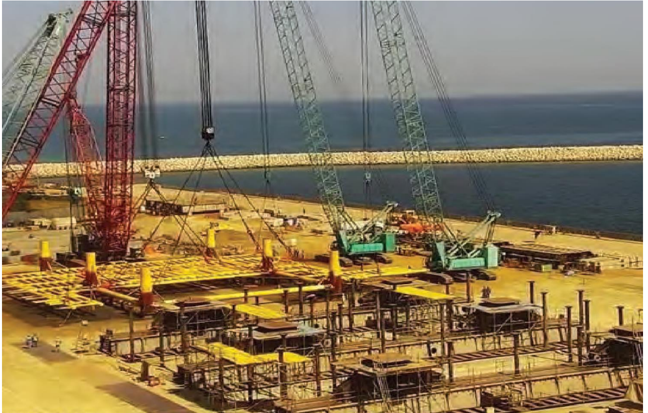
Hasbah-II: Fabrication of Topsides, MFY Sohar
