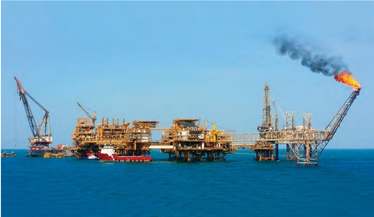
Bassein Development Project for ONGC. The scope included BCPA3 process platform, BLQ3 Living Quarters platform, BH wellhead platform, 12 km pipelines, bridges and modifications at BPA complex.
