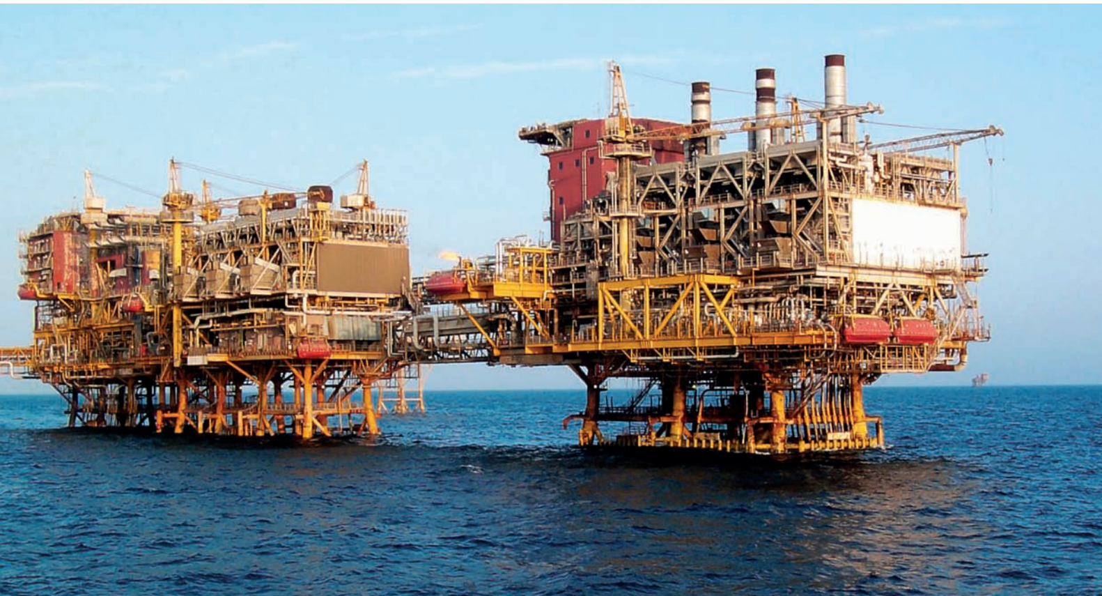
Booster compressor platform with an interconnecting bridge executed for Oil & Natural Gas Corporation (ONGC) in South Bassein Gas Fields off India's west coast. This project won the 'PMI Distinguished Project Award' from Project Management Institute, USA
