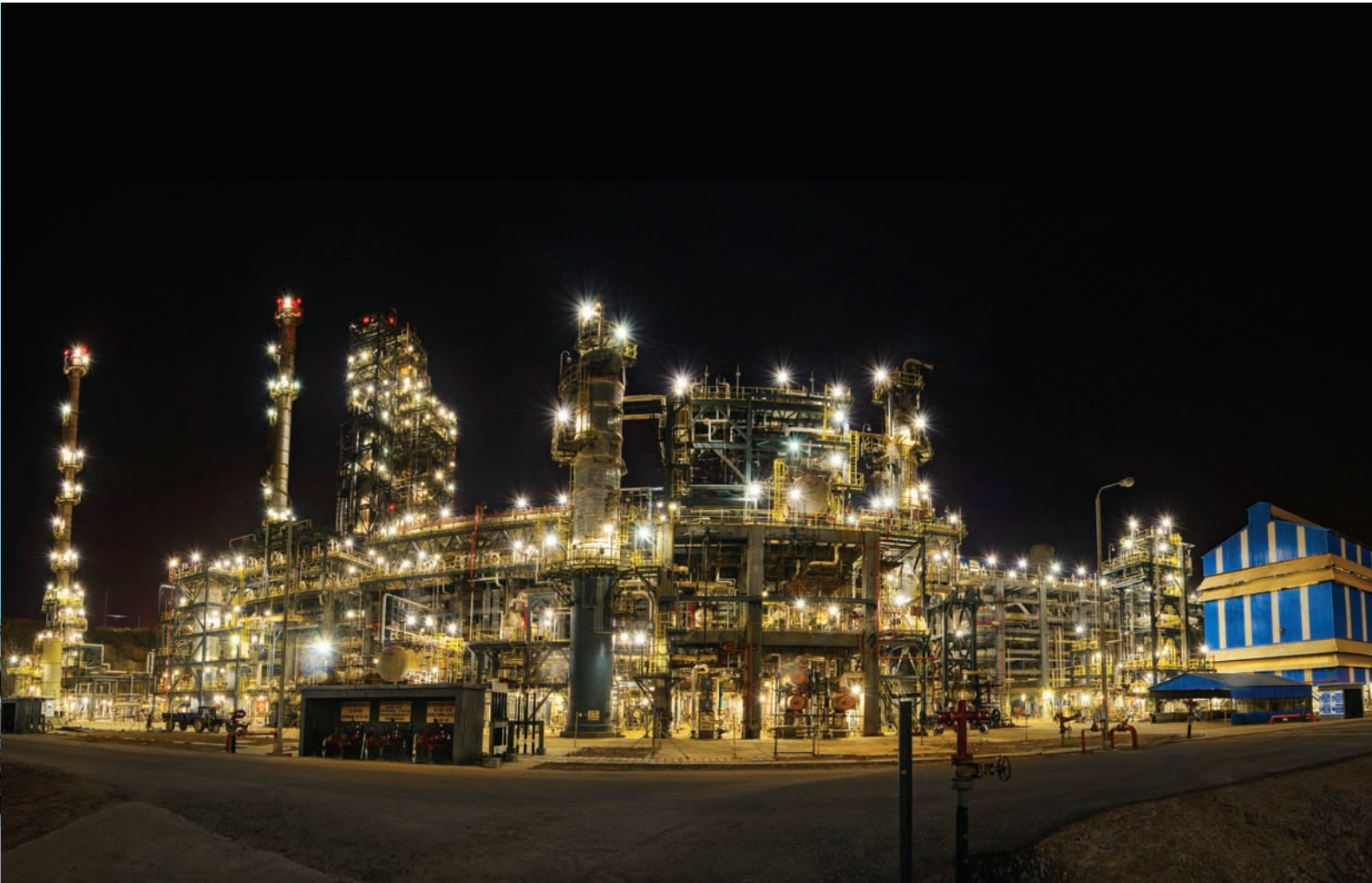
Aromatics Complex at Mangalore for ONGC - Mangalore Petrochemicals Limited
