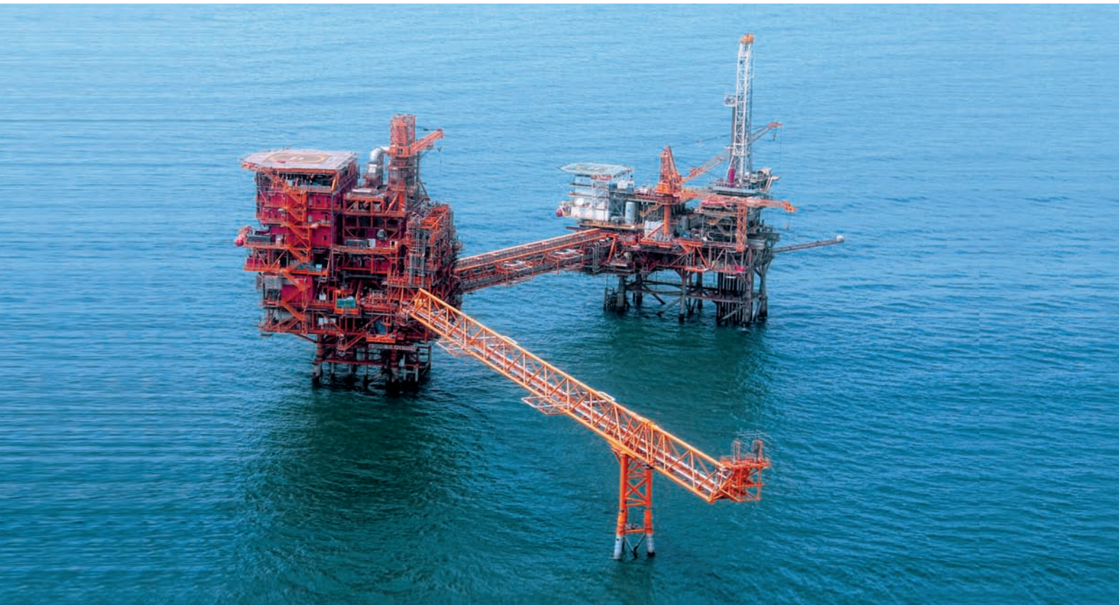
DDW1 Wellhead Platform & Process-cum-living Quarters Platform for GSPC, installed off India's east coast
