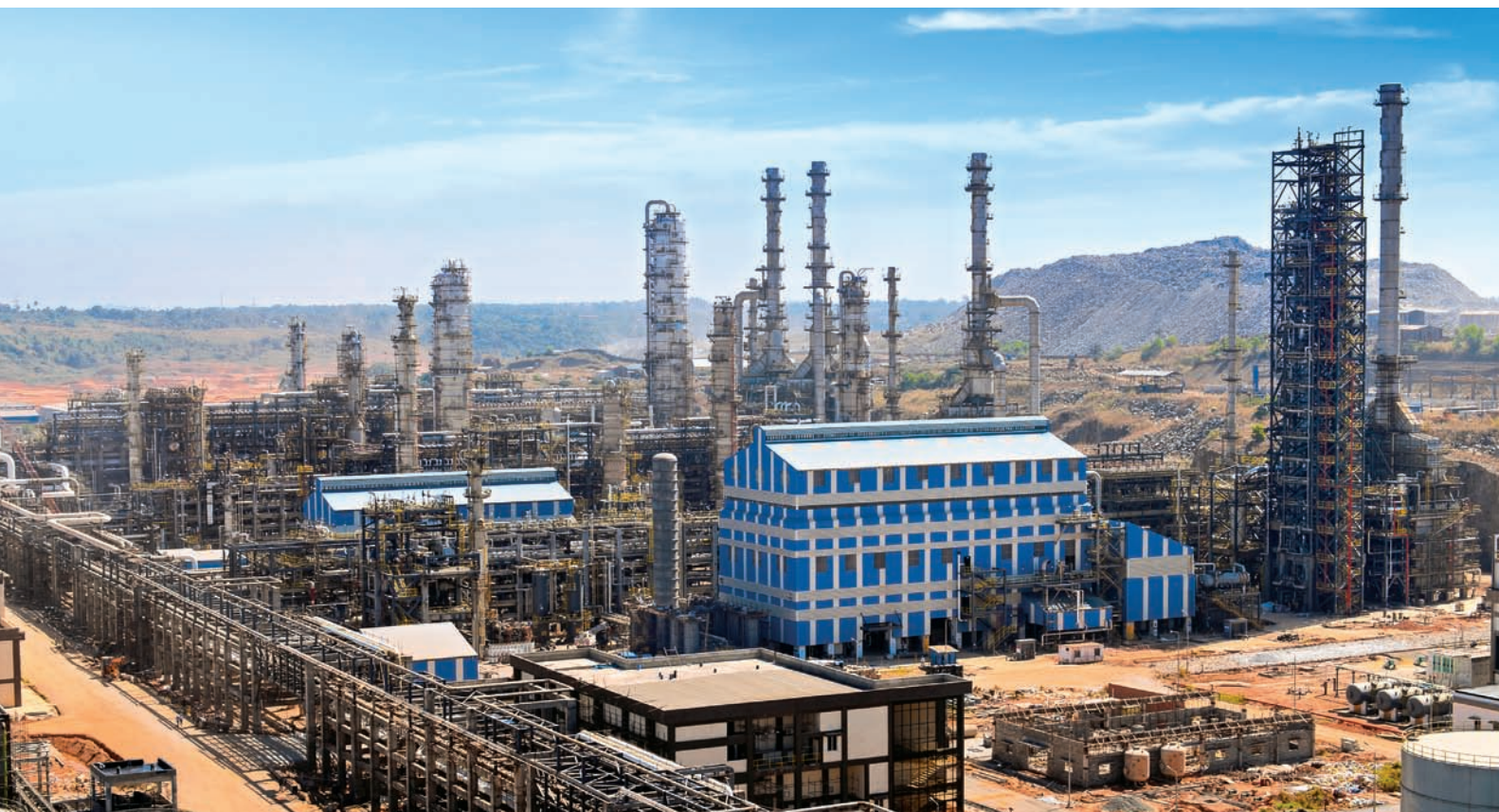
Mangalore Aromatic Complex for ONGC-Mangalore Petrochemicals Limited, India
